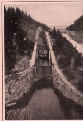
A TOURISTS' CANAL THAT CLIMBS NORWEGIAN HILLS The Bandal-Norddals Canal is a 10 1/4 mile link in the journey from Skien on the southern coast to Daleen in the Telemarken lake country. It rises 187 feet in seventeen locks. Here by the Vrangfos tourists are advised to get out and walk.
