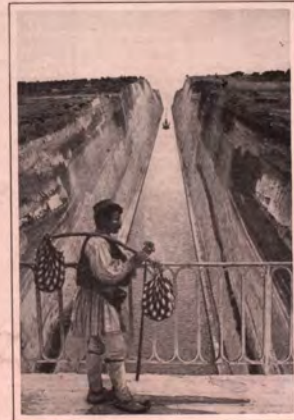
THE CORINTH CANAL—AN UNPROFITABLE FEAT Nero and the French both started to dig at Corinth and both gave it up. Greeks finished the canal in 1853. The banks are as high as Colchra would be if the Panama Canal were cut down to sea level. It is dangerous and little used by big ships.
